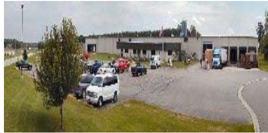
Lakeland Mills Inc., Edmore Industrial Park
